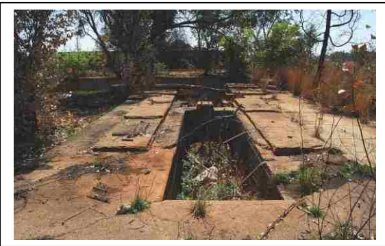
Fig. 3 Boiler plant foundations.
