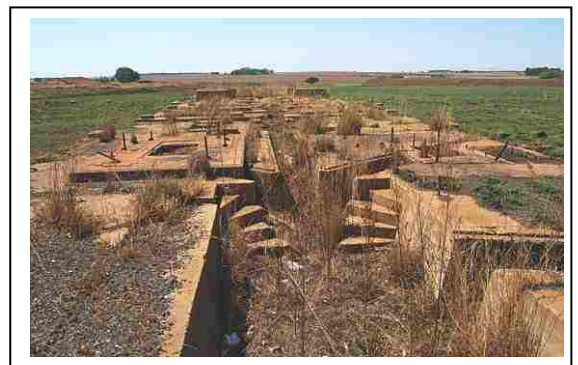
Fig. 8 Ball mill plant foundations.
