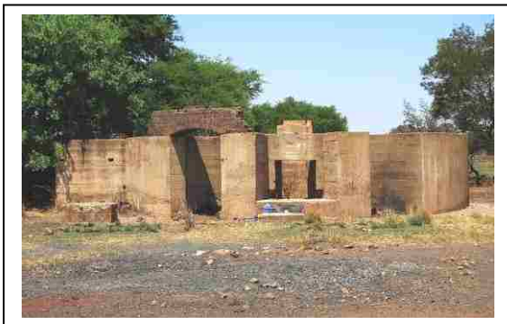
Fig. 5 Presumed Godfrey roaster foundations.
