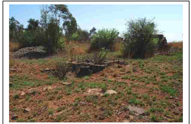
Fig. 14 Concentration Plant wheel pit and office foundations in foreground.
