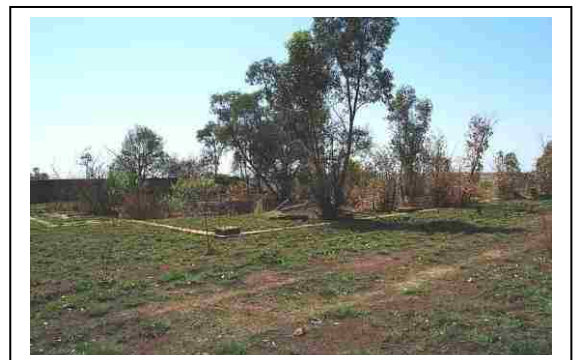
Fig. 6 Boiler plant external wall foundations.
