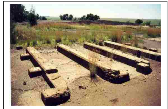
Fig. 2 Part of the concentration plant foundations.
