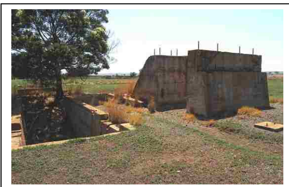
Fig. 7 Secondary crusher foundations.
