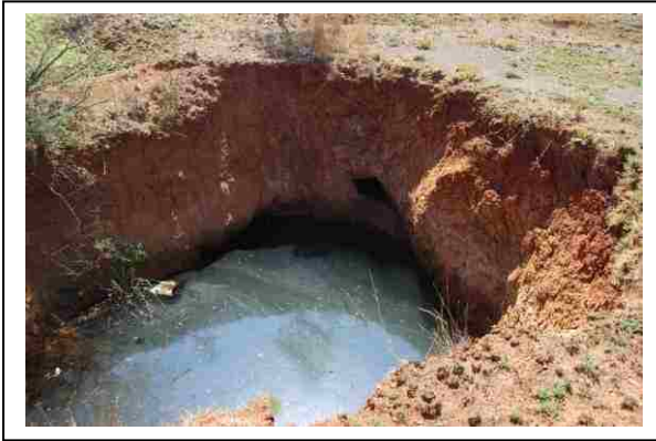
Fig. 9 Collapsed upper stope near winze E2.
