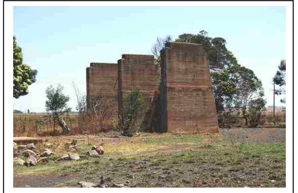
Fig. 12 Blast furnace foundations.
