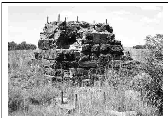
Fig 19 Blake jaw crusher foundation in 2008. 18
